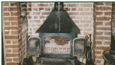
It has been shown in tests that the thatch adjacent to the chimney can reach 85% of the flue gas temperature after only one day of continuous use. The critical temperature of 200°C can be achieved and sustained with relative ease.
